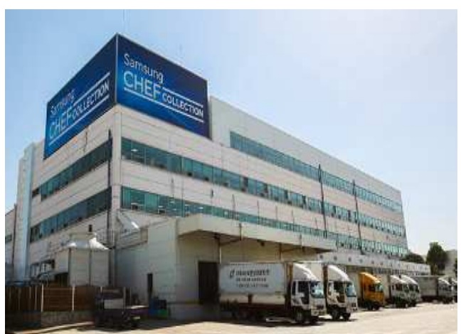
Figure 40. SEC's Gwangju plant (HA)
