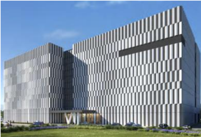
Figure 11. Dongtan data center (opened in Jan. 2023)
