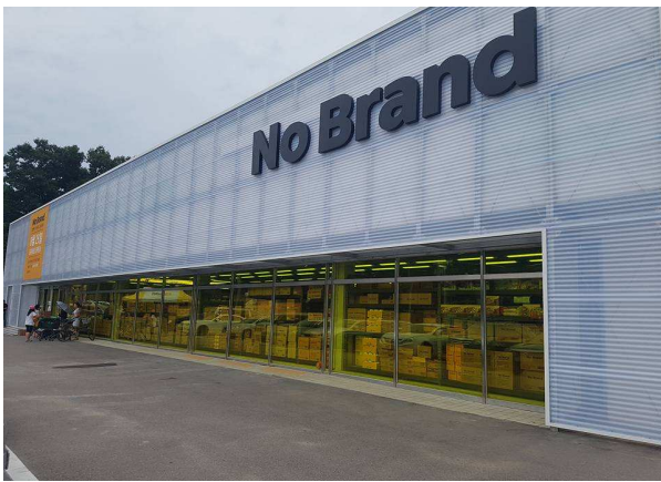
Figure 1. Exterior of No Brand store in Yongin (converted from Everyday)
