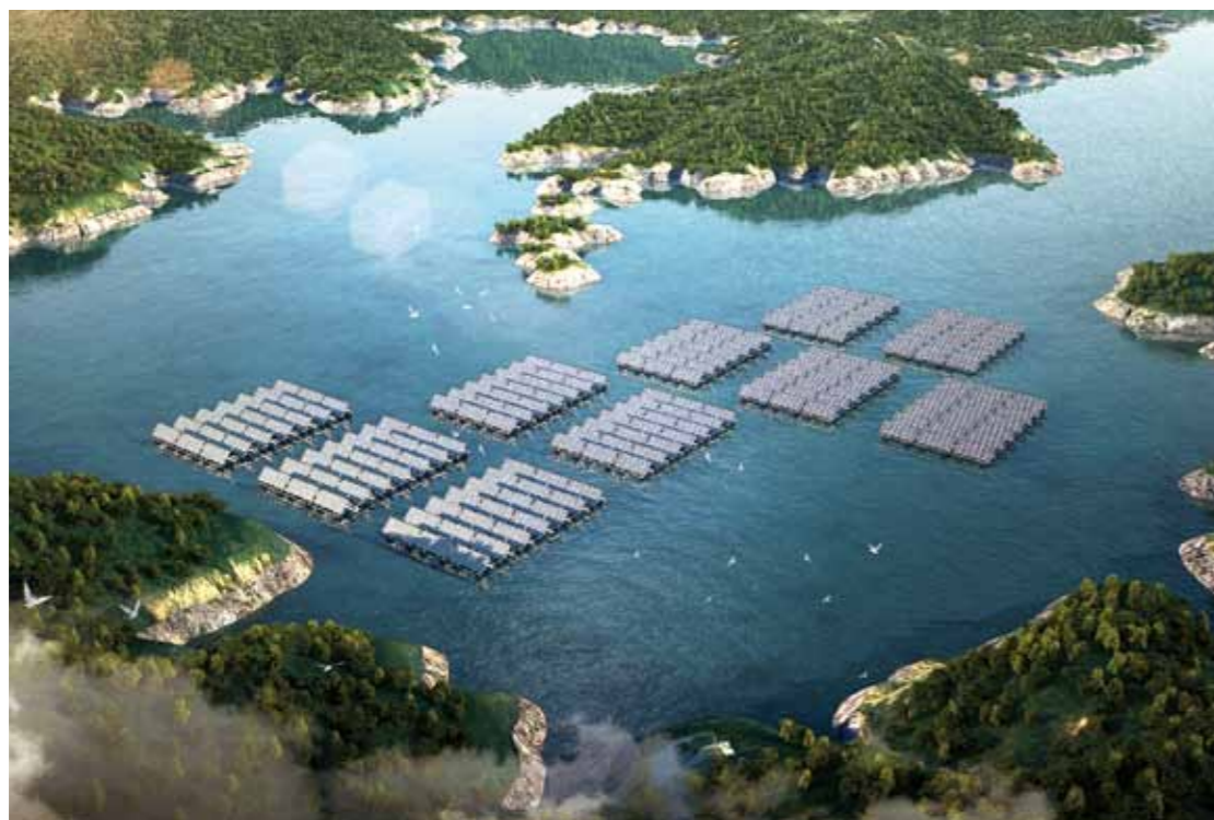
Partial bird's eye view of the Floating Solar Power Plant on Hapcheon Dam
